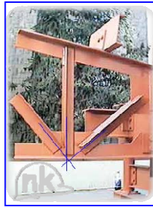
Fig. 9. Truss connections
