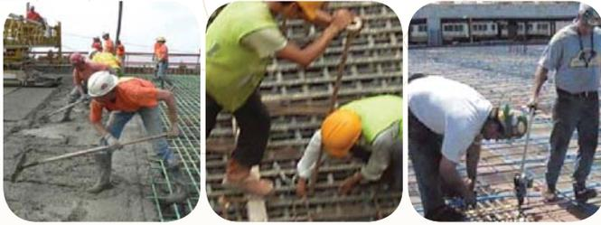
Figure 8: Left - 'bull-floating' with an awkward posture. Centre - squatting and wire binding rebar. Right - bending down and wire binding versus standing up and wire binding, using a mechanical aid.
