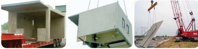
Figure 13. Left - transportation of unit. Centre - lifting of unit. Right - lifting of tilt-up slab.
