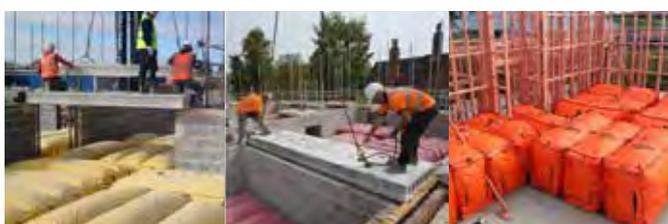
Fig. 6. Air-bags in general, concrete, and timber construction
